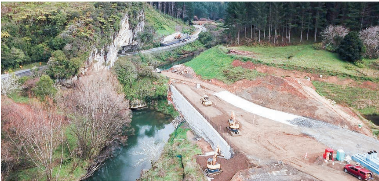
Awakino Tunnel Bypass - The tunnel on the left will be bypassed by two bridges across the Awakino River.
